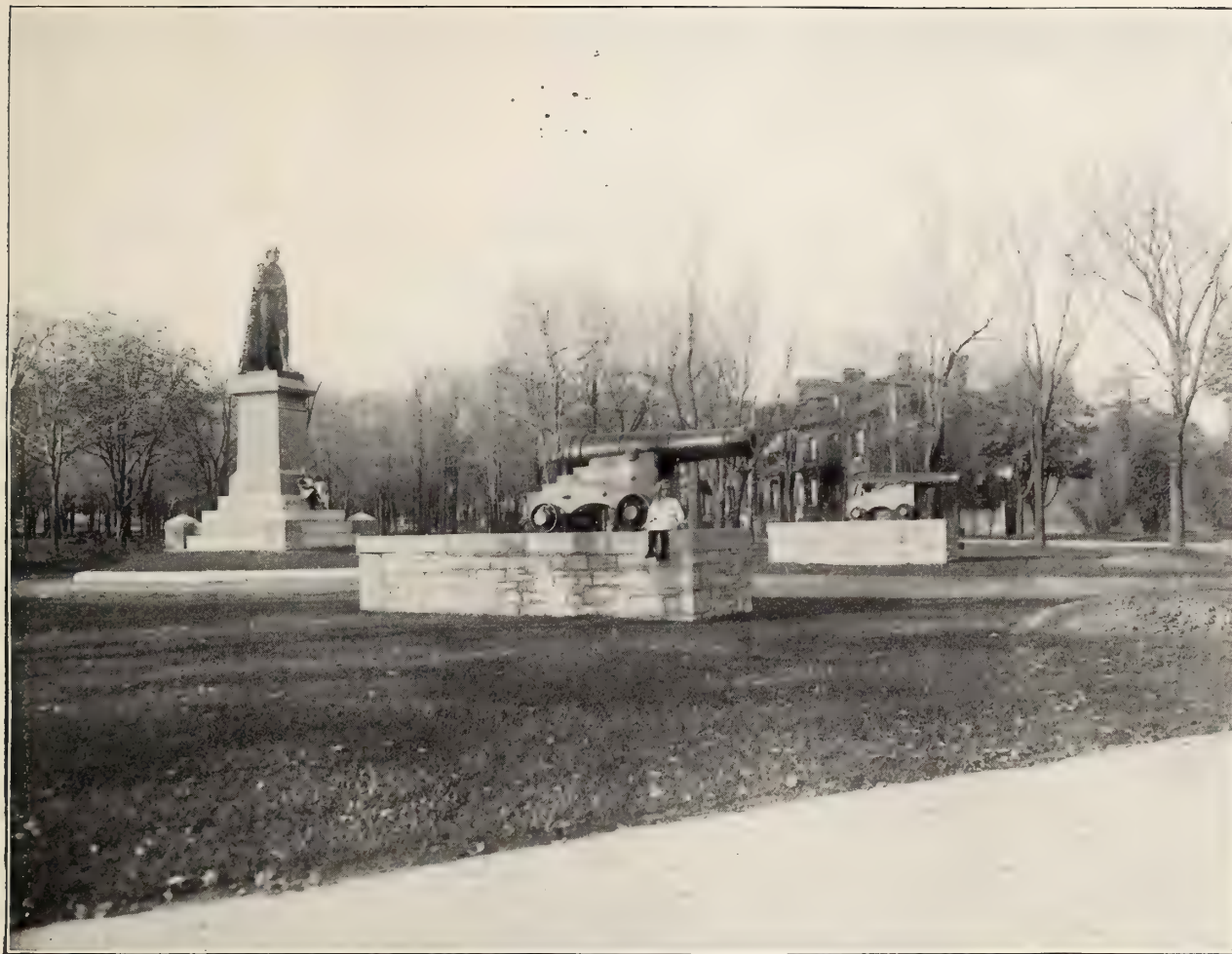
Entrance to City Park and Sir John A. Macdonald Monument.
